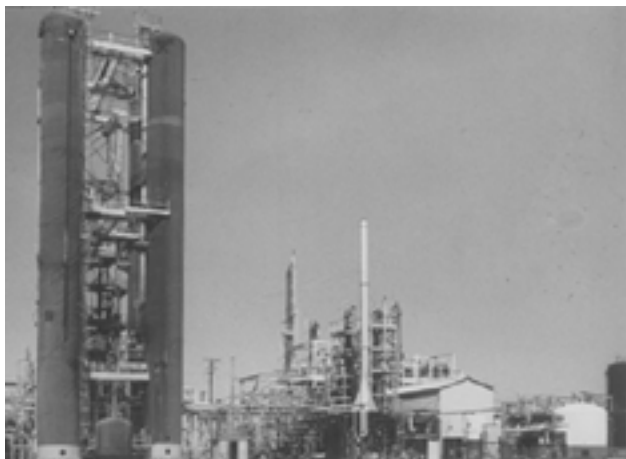
Fig. 2-50. The first three steps of VX nerve agent production were completed in these structures at Newport, Indiana. The technological level of chemical engineering needed to make this agent is vastly more complicated than that required to make mustard and phosgene during the World War I era. Photograph: Chemical and Biological Defense Command Historical Research and Response Team, Aberdeen Proving Ground, Md.
