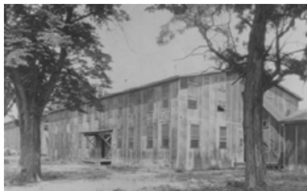
Fig. 2-15. The first temporary Chemical Warfare School building at Edgewood Arsenal, Md., shortly after the end of World War I. The school was later moved to a permanent structure. Photograph: Chemical and Biological Defense Command Historical Research and Response Team, Aberdeen Proving Ground, Md.
